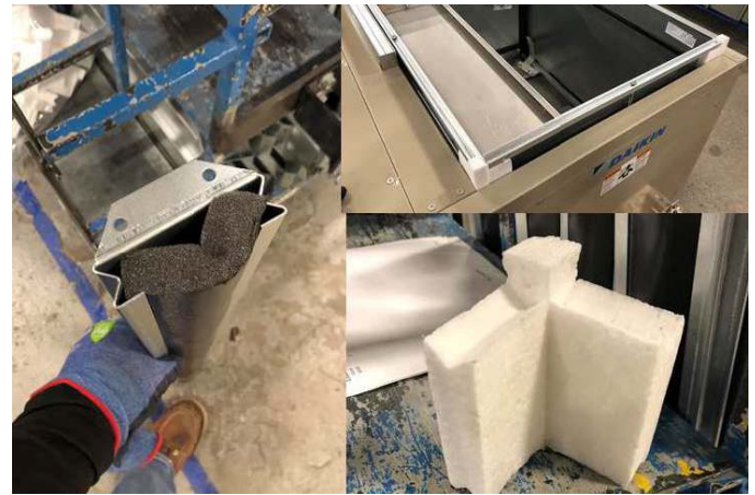
Figure 7: Shipping Braces
